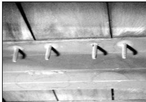
Figure 3-5. Decking Board Screws in Frame
